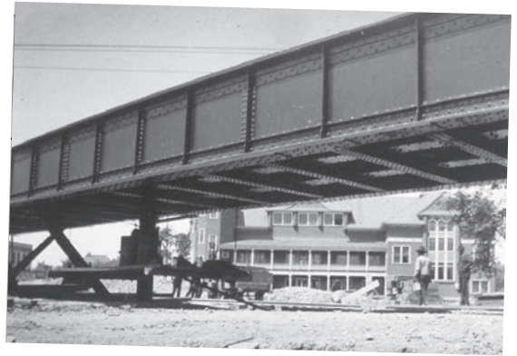
Track elevation nearing completion, looking north on Irving Park Blvd at Keeler (Irving Park Club in bkgd), 1898
